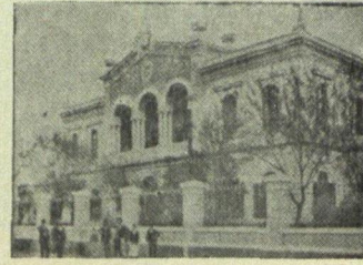
Hospital San Roque — Buenos Aires
